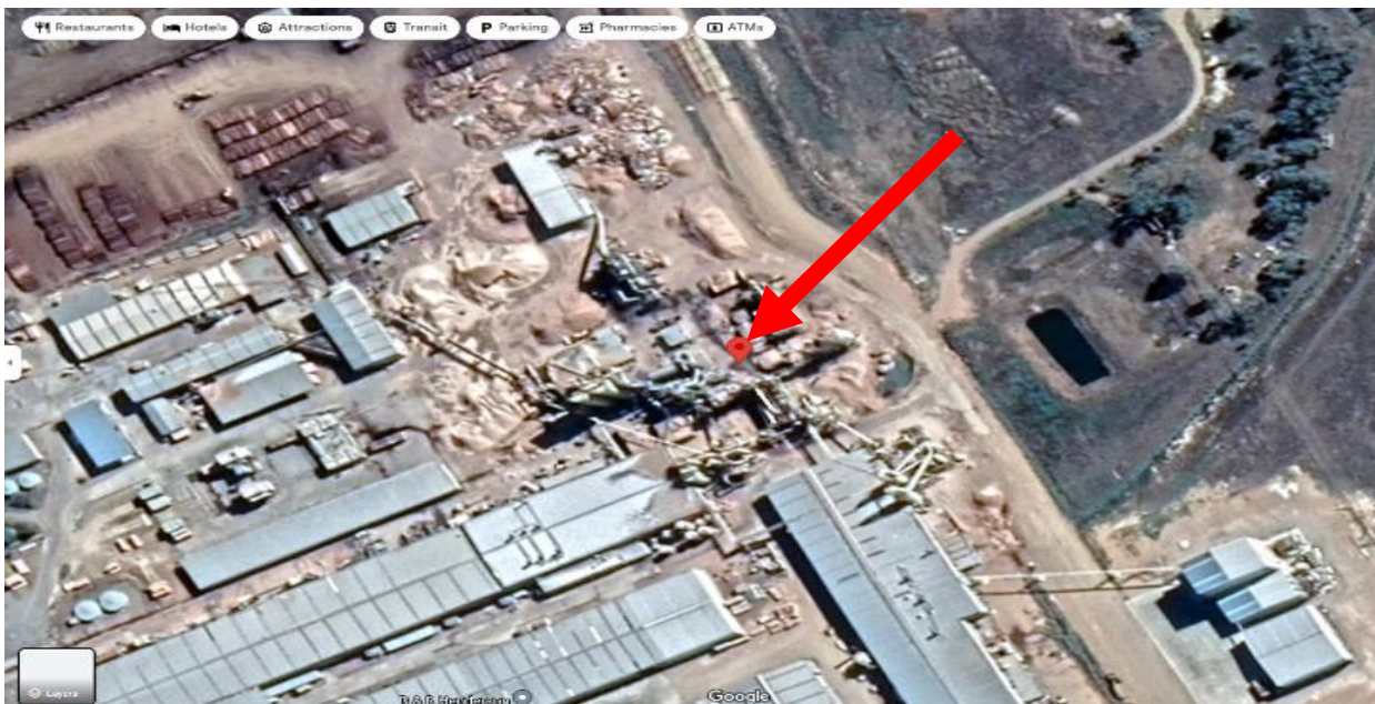
Figure 6: Aerial view of Facility with proposed location of the WESP and Heat Plant (Source: Application)
